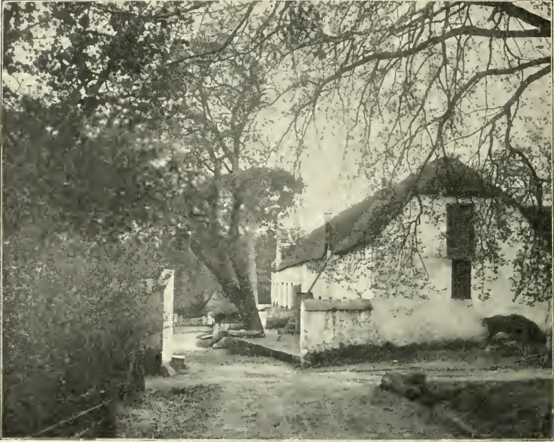
AN OLD BOER HOMESTEAD IN THE INTERIOR OF THE TRANSVAAL.
