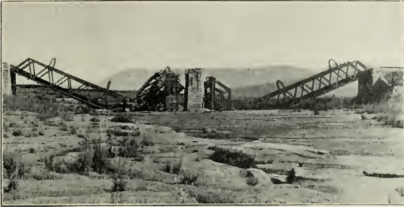
THE RAILWAY BRIDGE AT WASCHBANK (NATAL), BLOWN UP WITH DYNAMITE BY THE BOERS.
