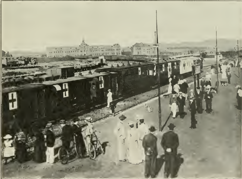
ONE OF THE NETHERLANDS SOUTH AFRICAN RAILWAY COMPANY'S TRAINS TRANSFORMED INTO AN AMBULANCE-TRAIN. At the commencement of the war, the Netherlands South African Railway fitted up several railway-carriages for the conveyance of the wounded with beds, drug-stores, and compartments for re-dressing wounds. The last carriage in particular, the large white ambulance-carriage, was a master-piece that did great credit to the ingenuity of the railway-officials at Pretoria.
