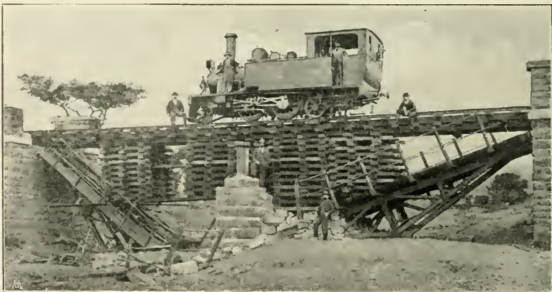
THE RAILWAY BRIDGE OVER THE SUNDAY RIVER (NATAL), REPAIRED BY THE TRANSVAALERS. The English repair bridges in the same manner, or else build a kind of bridge in the bed of the river. These are, of course, only make-shifts, and quite unable to resist the rapids, especially after the tropical rains, when the force of the current becomes exceedingly strong.
