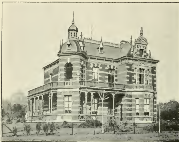
A PRIVATE HOUSE AT PRETORIA.
